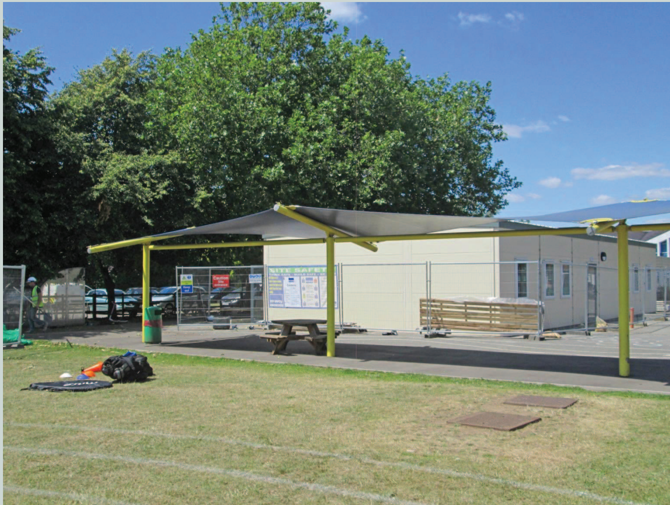
Fig 3 : Looking northwest showing new demountable unit and trees with a section of protective fencing
