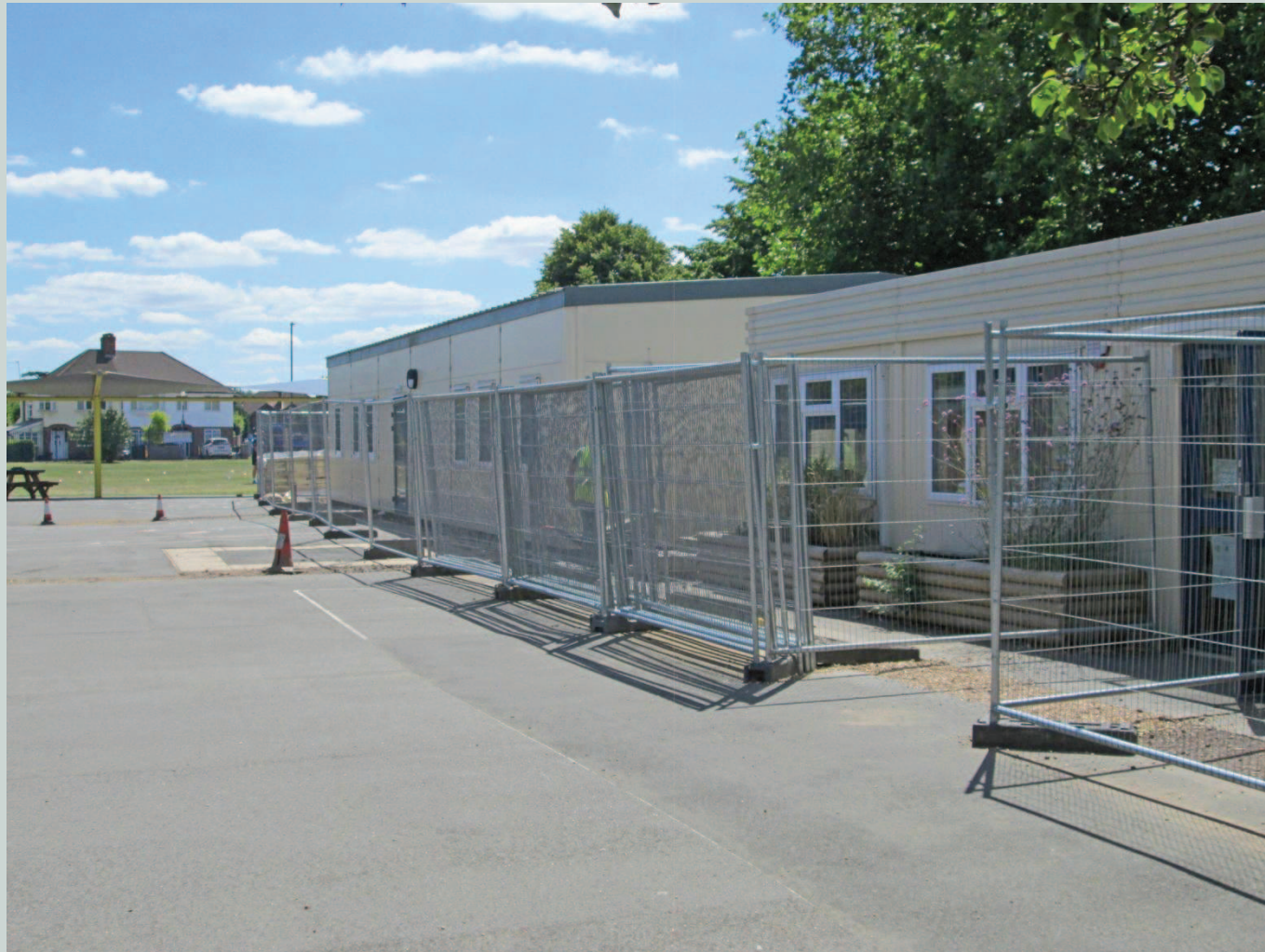
Fig 1 : Looking south from hard play area toward demountable unit under construction
