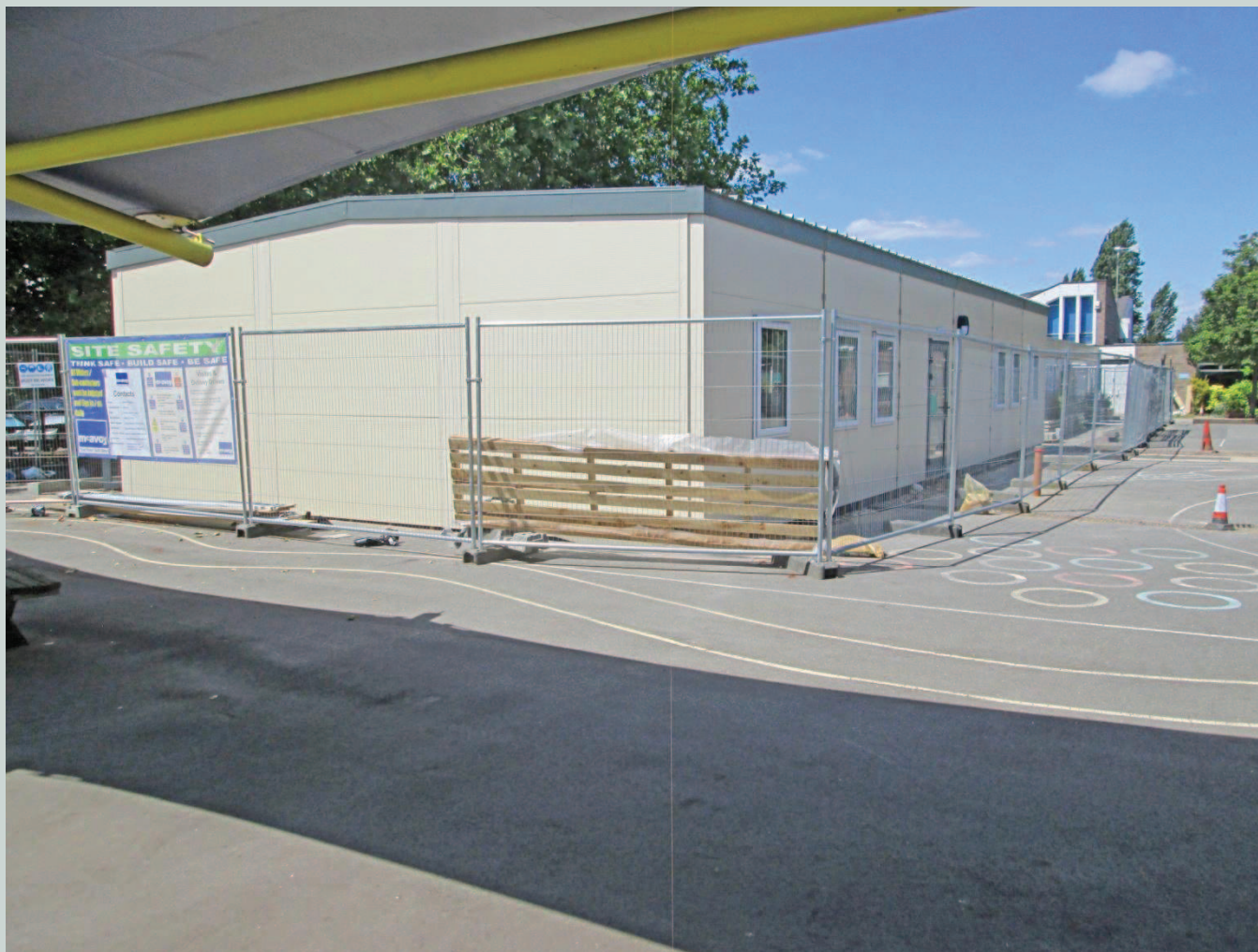
Fig 2 : View looking northwest toward demountable unit under construction
